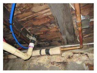
Observation #11.3: Water stains and damaged interior finishes were observed in many locations in the attic space.
