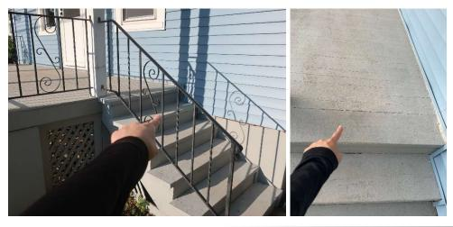
Observation #5.5: A crack was observed between that rear side stair and the building wall. The stair appears to be unlevel.
