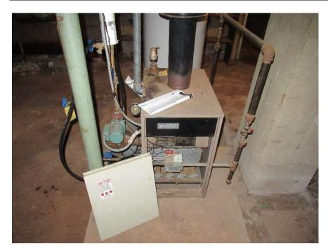
Heating energy source(s): Natural gas Primary Heating system: Boiler Distribution system: Hydronic baseboard
