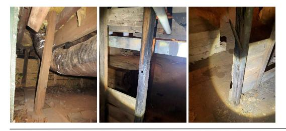
Observation #4.4: Many horizontal beams/joists in the crawlspace were damaged. Some of the beams appeared to be damaged by wood destroying insects and some of the beams appeared to be damaged by fire. Some of the beams have significant cracking. Multiple connections between the beams and the vertical supports were improper.
