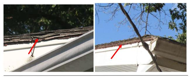
Observation #6.2: Obstructed/clogged gutter. The gutters around the building appear to be clogged by leaves and debris.
