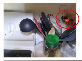
Observation #6.3: The GFCI in the bathroom was not tripping when tested.
