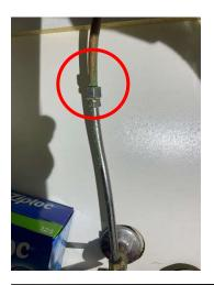
Observation #5.2: The hole in the wall is too large for the drainage pipe under the bathroom sink. A gap was visible.
