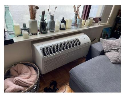
Heating and cooling energy source(s): Electricity Primary Heating system: Packaged Terminal Air Conditioner (PTAC) Cooling equipment type: In-wall air conditioning unit
